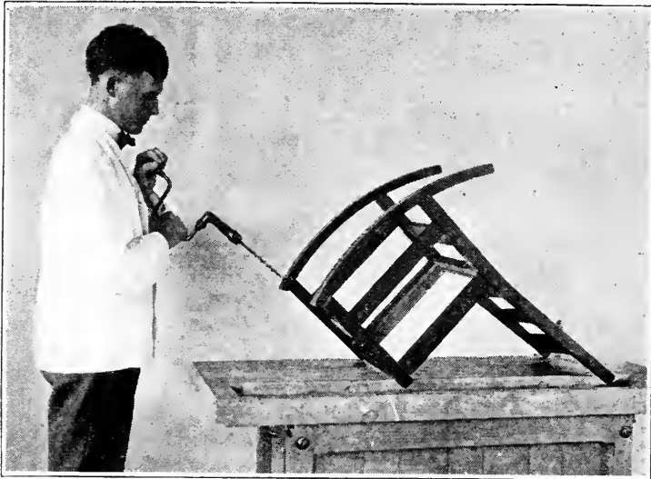
FIG. 402. BORING FOR DOWELING.
